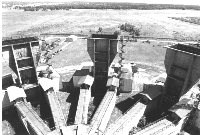
Fig.8.31. Fan station of central ventilation, Sieroszowice mine (after Wacławik et al, 1996)
