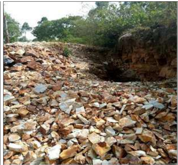
F. Deep Open Pit and Dumped Debris
