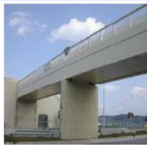
Fig. Pedestrian Bridge in Okinawa, Japan made of Hybrid Composite.
