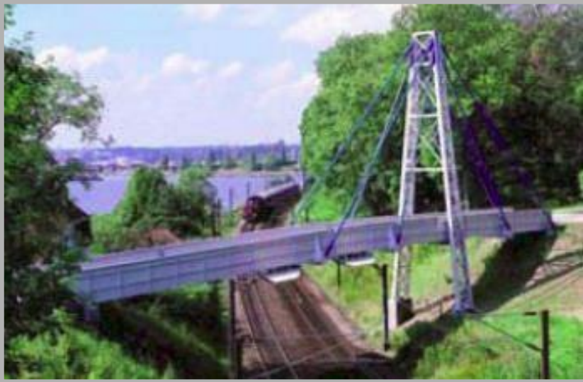
Pedestrian bridge in Denmark, 130 feet long (1997)
