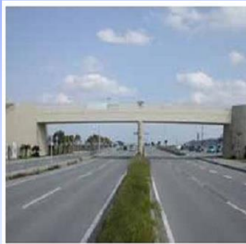
Fig. Pedestrian Bridge in Okinawa, Japan made of Hybrid Composite.
