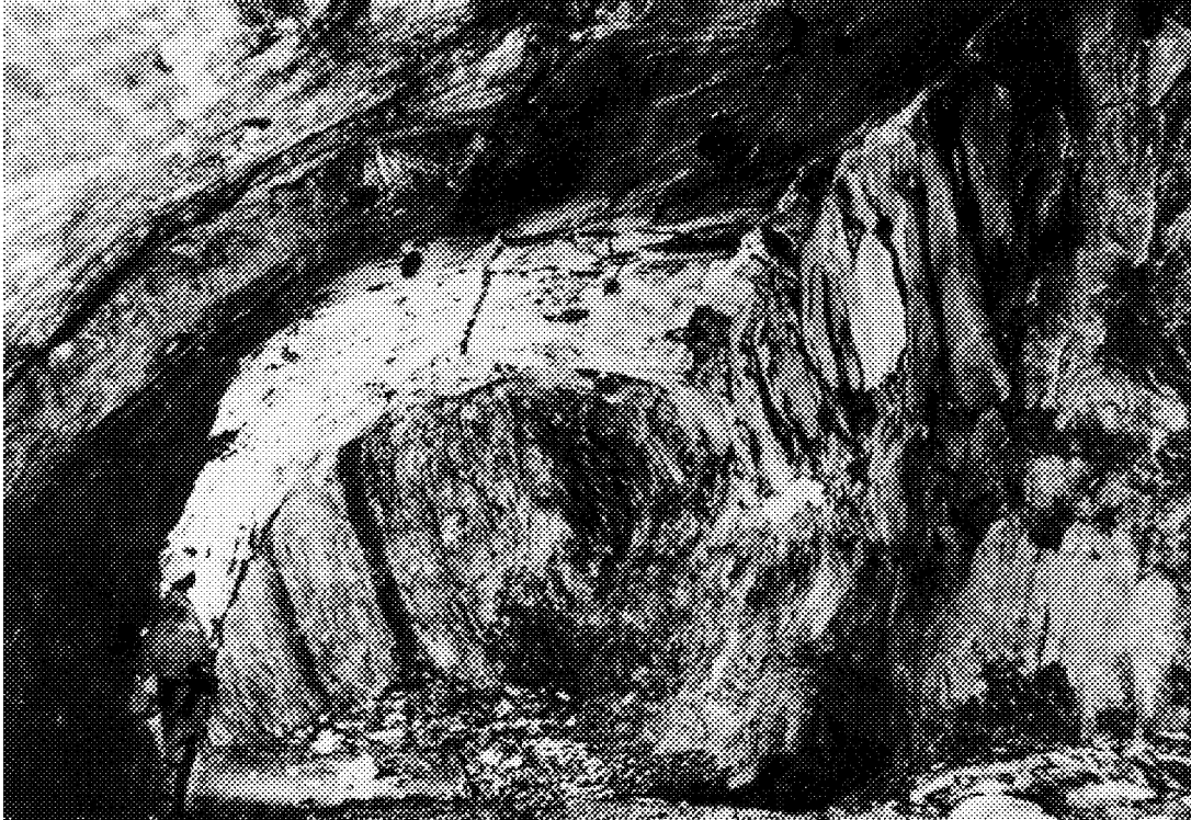
Figure 10.14: Spalling around a tunnel in massive quartzite at a depth of 2,700 m below surface in a South African gold mine. Photograph provided by Mr David Ortlepp.
