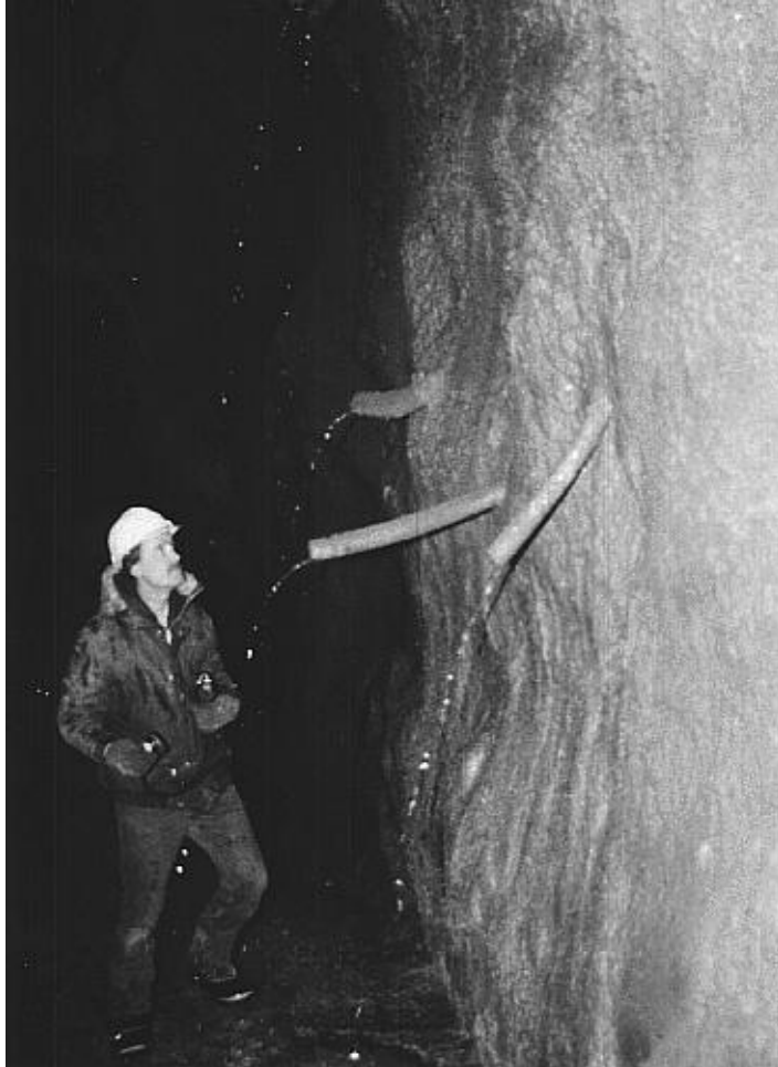
Figure 15.9: Plastic pipes used to provide drainage for a shotcrete layer applied to a rock mass with water-bearing joints.
