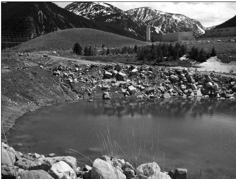
Figure 3. Percolation pond used for disposal of treated mine water. Treated water is discharged to the percolation pond where it infiltrates subsurface to ground water, mixes and eventually flows to surface water. The percolation ponds at both mines are NPDES-permitted outfalls. (DEQ photo)
